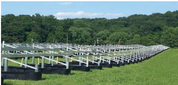
Courtesy GameChange Racking
