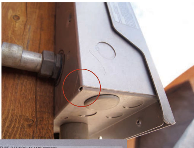
This NEMA 3R combiner box is rainproof, but not rain- or watertight. The weep hole allows water to drain from the box.
