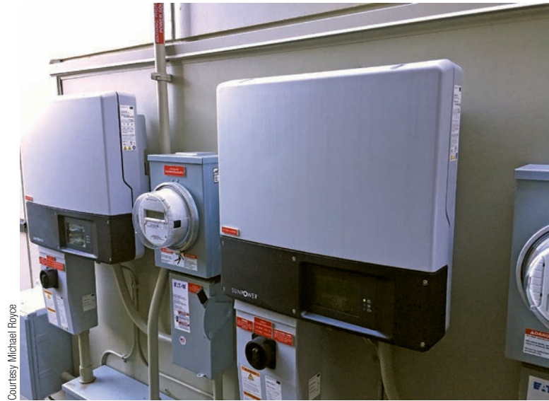
Each home has its own PV array, inverter, and production meter. Inverters are SMA Sunny Boy 3800TL-US models rebranded by SunPower.
