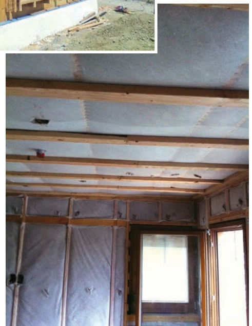
Left: Two-by-four framed walls are combined with 9.5-inch I-joist trusses. The cavities filled are filled with dense-pack cellulose insulation, creating R-45 walls.
