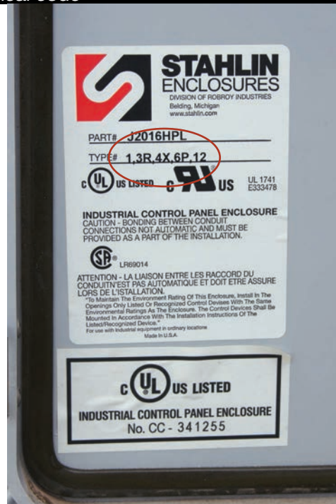
This combiner box has multiple NEMA ratings, including 4X. Note the gasketed cover, which makes it rain/watertight.
