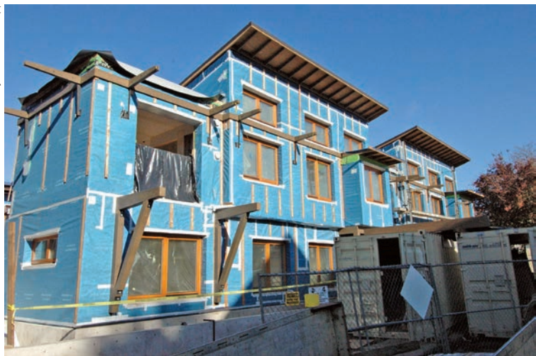
The moisture and air barrier is SIGA Majvest woven polyolefin, which helps keep air leakage under 1.00 ACH 50.
